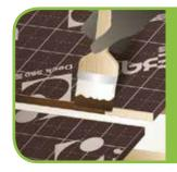
When cutting plywood, protect flat ends with paint, such as Teknol JRL (Finland), or a sealant to prevent penetration of moisture (swelling).
